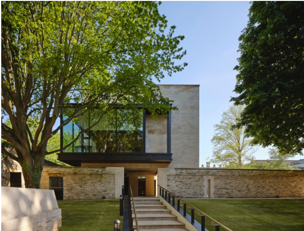
St John's College Library and Study Centre by Wright & Wright Architects © Dennis Gilbert
