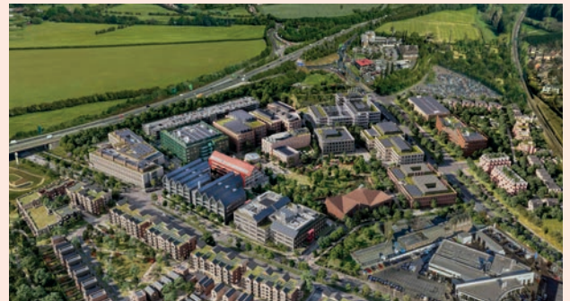
Aerial view of Oxford North site
